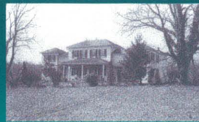
Boyle House at 4452 MacArthur Boulevard—on the site of Riverside Hospital.
