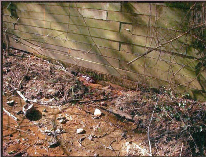
Seepage under Canal View ret. wall
