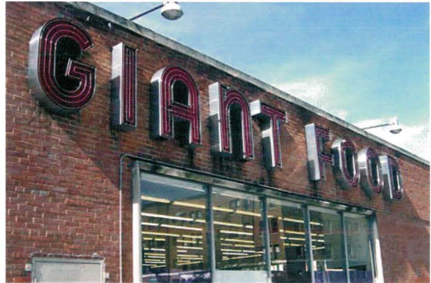
Photo 6: Closeup of the Giant Food facade
