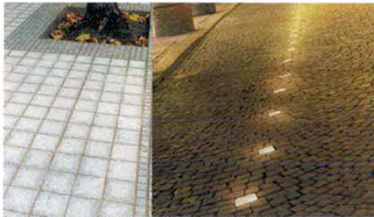
Porte Cochere: Granite paving with LED Lighting
