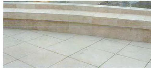
Outdoor Restaurant: Hanover Pavers and Wall Cladding
