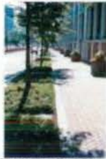
Continuous Tree Pit for L Street
