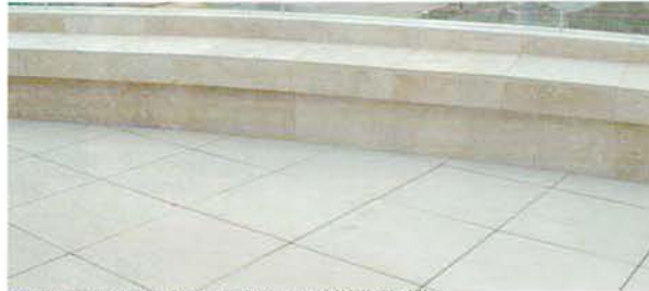
Outdoor Restaurant: Hanover Pavers and Wall Cladding
