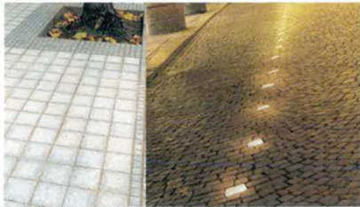
Porte Cochere: Granite paving with LED Lighting
