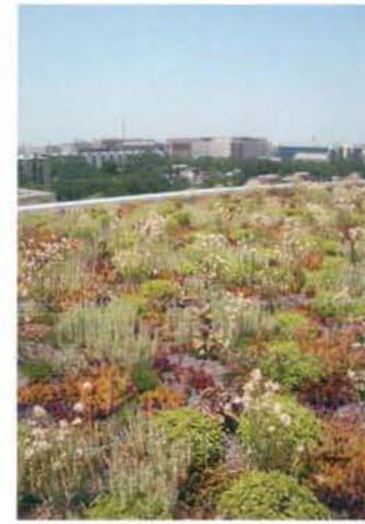
EXTENSIVE GREEN ROOF
