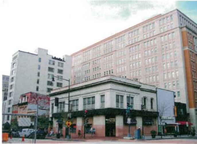
1. VIEW OF SITE - SOUTHWEST CORNER 10TH & F STREETS
