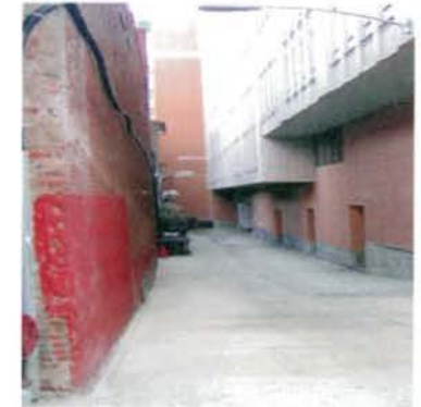
3. F STREET ALLEY LOOKING SOUTH
