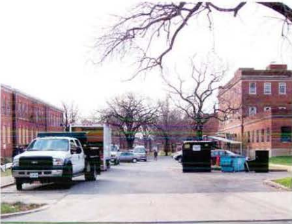
10. FIRST STREET LOOKING SOUTH
