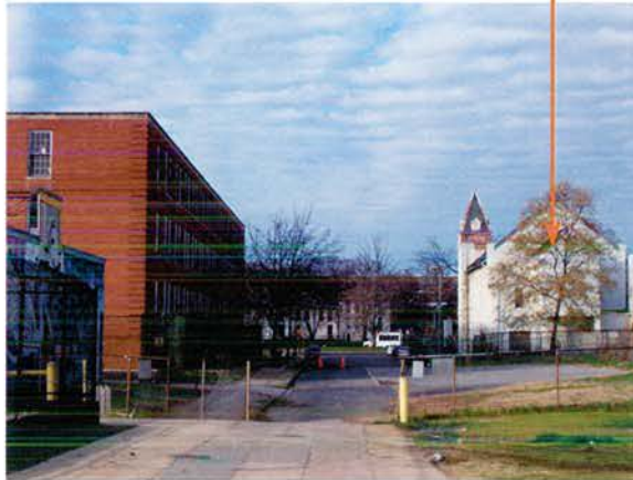
16. H STREET LOOKING WEST
