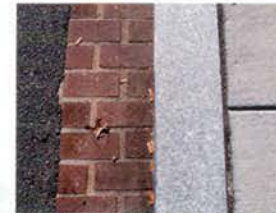
DC CURB/GUTTER/CONCRETE PAVING
