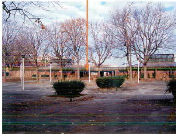
17. VIEW OF RECREATION CENTER FROM EYE STREET
