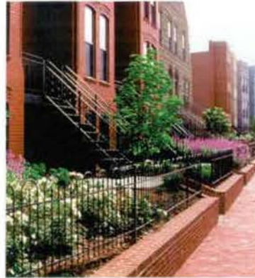
REBUILT BRICK RETAINING WALL
