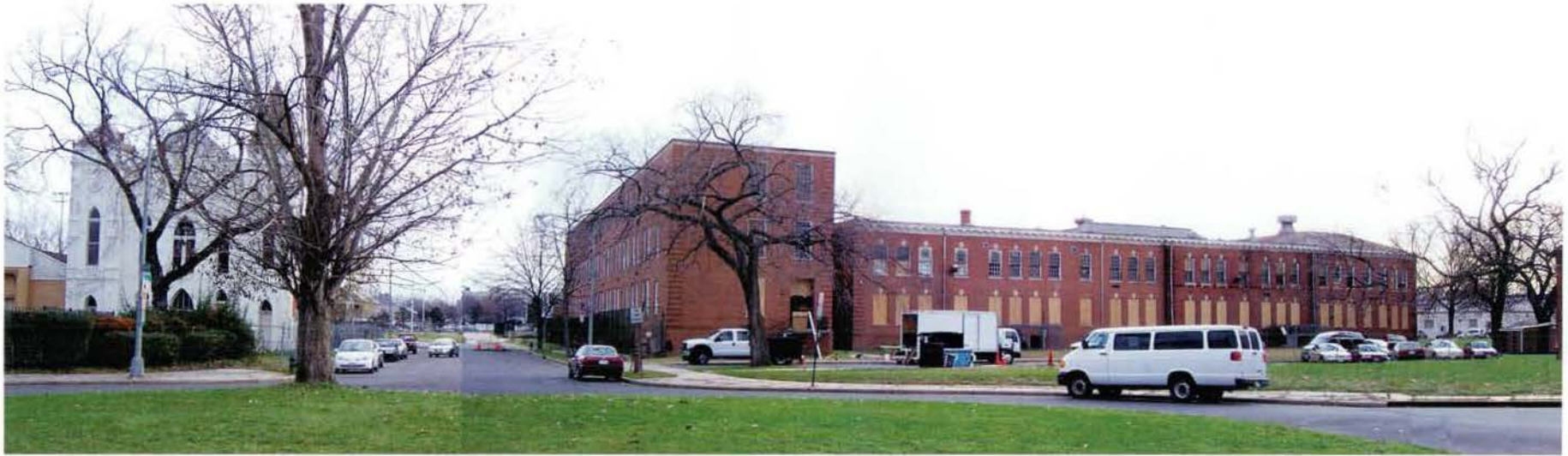
3. CORNER OF DELAWARE & H STREETS LOOKING EAST
