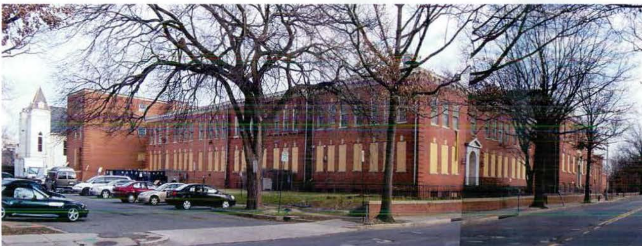
2. CORNER OF EYE & FIRST STREETS LOOKING NORTHEAST
