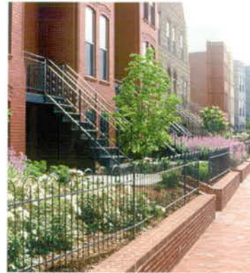
REBUILT BRICK RETAINING WALL
