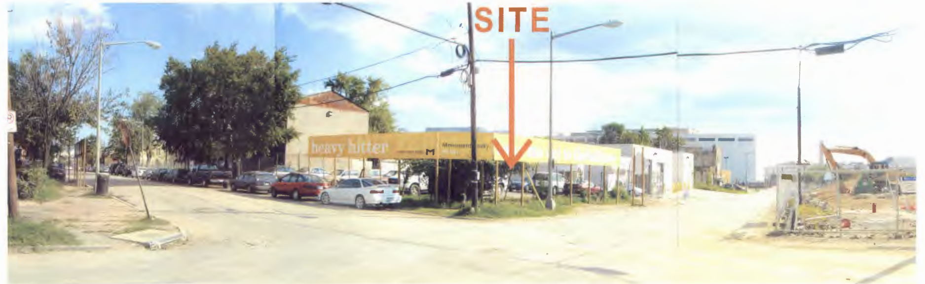
6. N & HALF STREETS INTERSECTION LOOKING EAST
