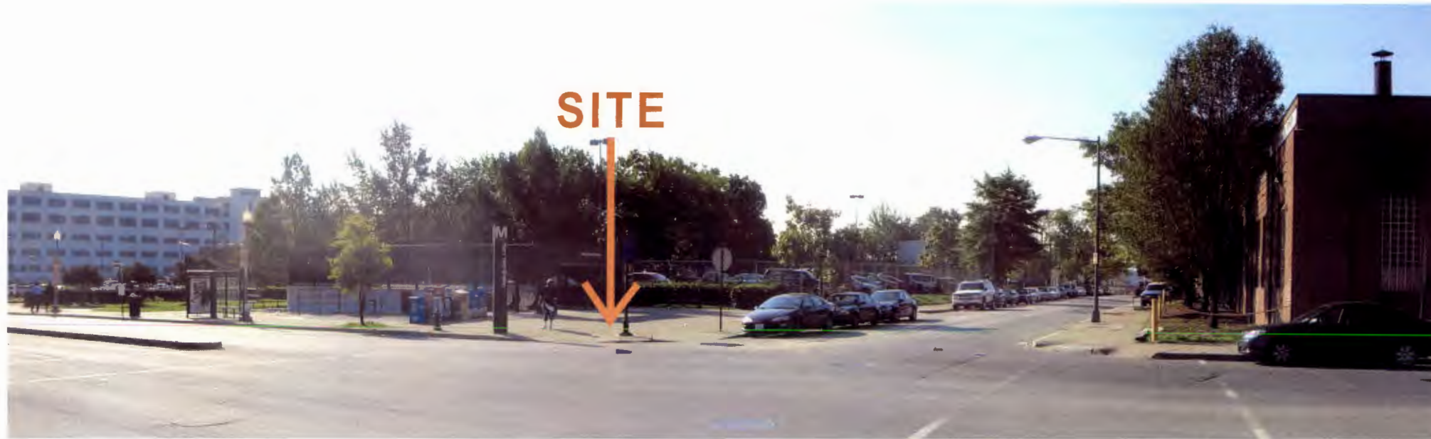
1. M & HALF STREETS INTERSECTION LOOKING SOUTH
