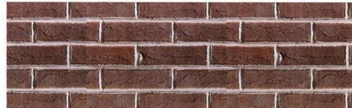
BRICK AT UPPER RESIDENTIAL UNITS
