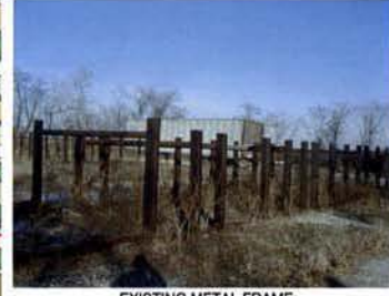
EXISTING METAL FRAME
