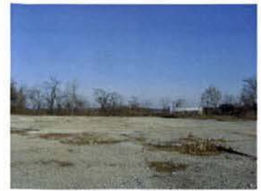
CONCRETE PAVED STOCKYARD
