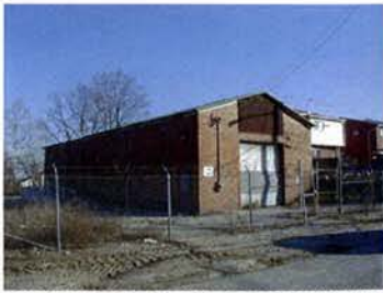
CHAINLINK FENCE AND EXISTING BRICK STRUCTURE
