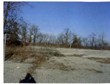
CONCRETE PAVED STOCKYARD
