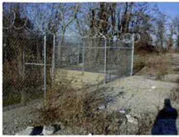
CHAINLINK FENCE AND RAZOR-WIRE
