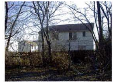
REAR OF DUPLEX AND WOODEN FENCE ADJACENT TO SITE
