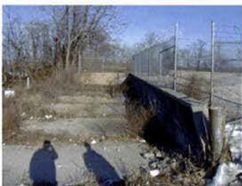
CONCRETE RETAINING WALL AND CHAINLINK FENCE
