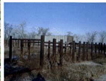
EXISTING METAL FRAME
