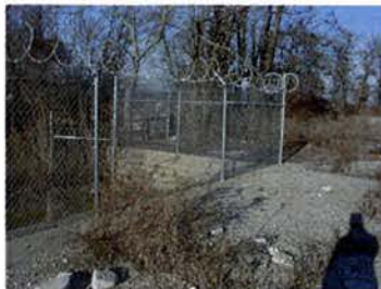
CHAINLINK FENCE AND RAZOR-WIRE
