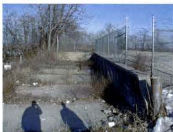
CONCRETE RETAINING WALL AND CHAINLINK FENCE
