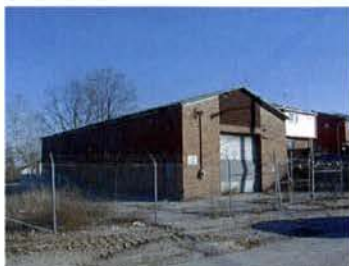
CHAINLINK FENCE AND EXISTING BRICK STRUCTURE
