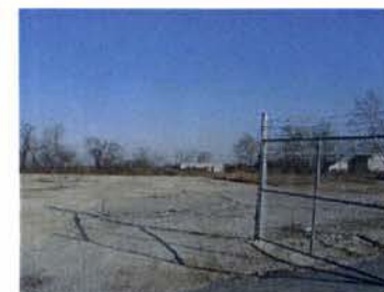
CONCRETE PAVED STOCKYARD
