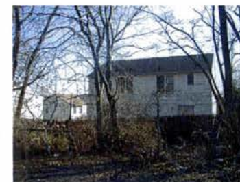
REAR OF DUPLEX AND WOODEN FENCE ADJACENT TO SITE
