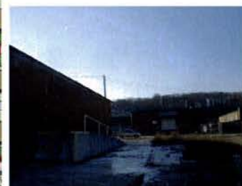
EXISTING BRICK STRUCTURE
