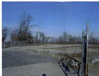
CHAINLINK FENCE AND CONCRETE PAVED STOCK YARD
