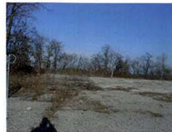
CONCRETE PAVED STOCKYARD
