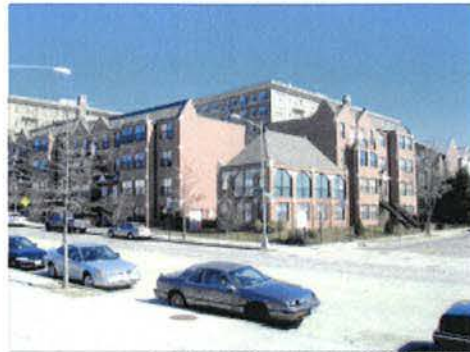
9. EXISTING BUILDINGS ACROSS FROM SITE
