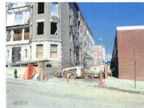
7. VIEW OF ALLEY FROM SOUTH SIDE
