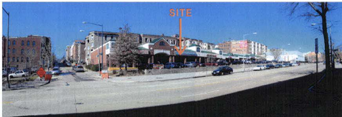
2. VIEW OF SITE - SOUTH SIDE
