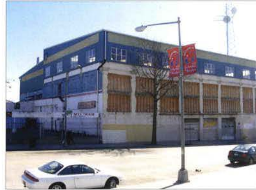
4. EXISTING BUILDING SOUTHEAST OF SITE
