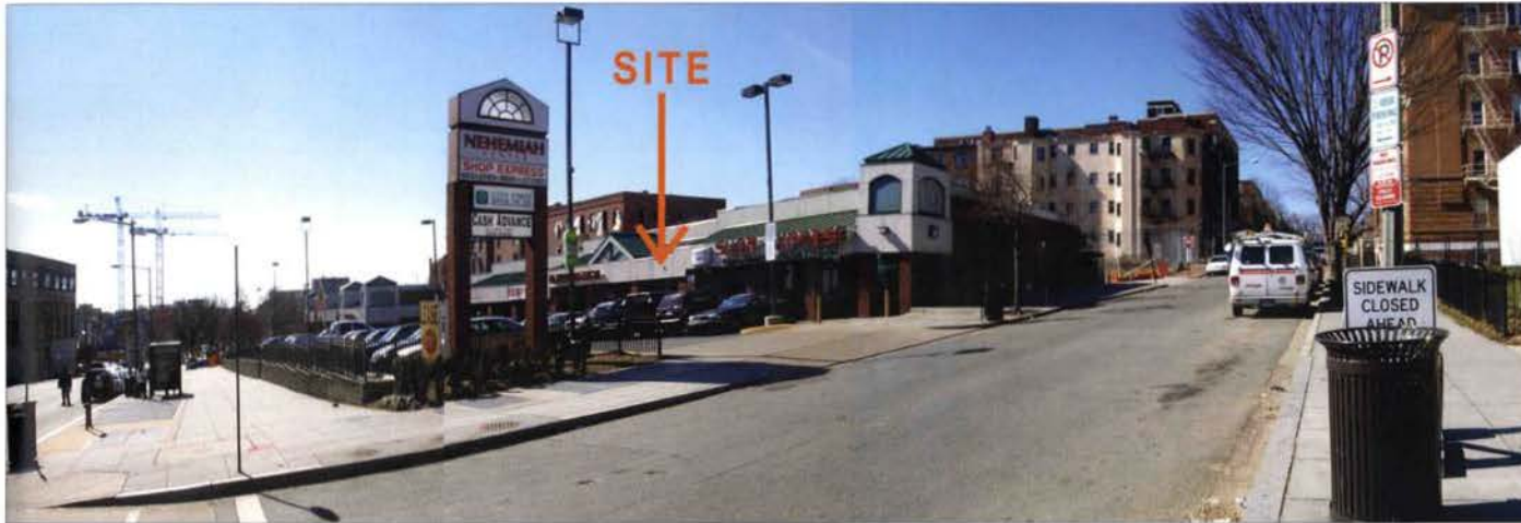
1. VIEW OF SITE - NORTH SIDE
