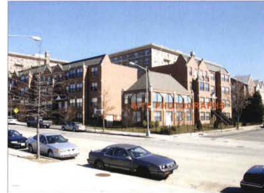
8. EXISTING BUILDINGS ACROSS FROM SITE
