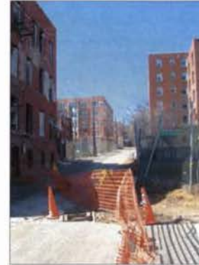
5. VIEW WEST THROUGH ALLEY
