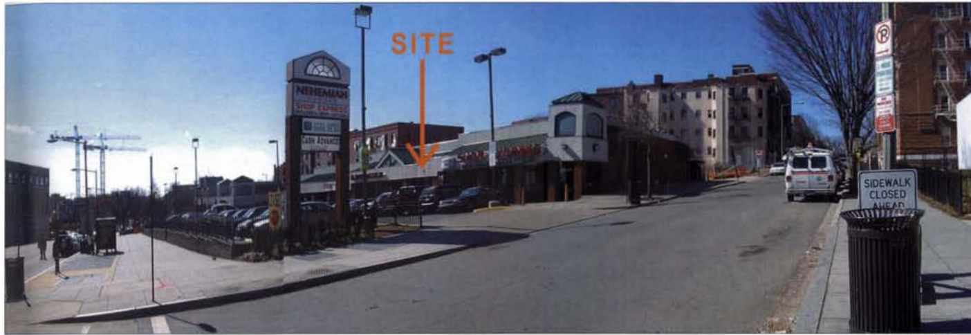
1. VIEW OF SITE - NORTH SIDE
