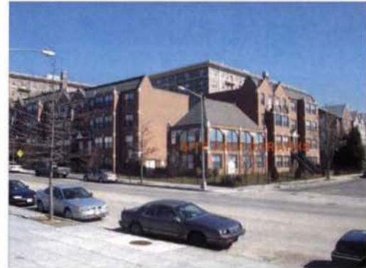
8. EXISTING BUILDINGS ACROSS FROM SITE
