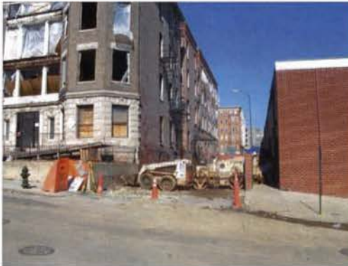
7. VIEW OF ALLEY FROM SOUTH SIDE
