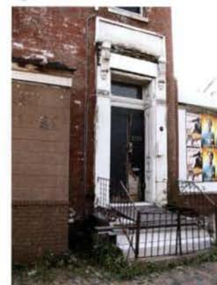
6 1100 6TH ST EXISTING HISTORIC STRUCTURE: FRONT DOOR DETAIL
