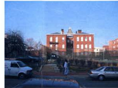
South facade from F Street
