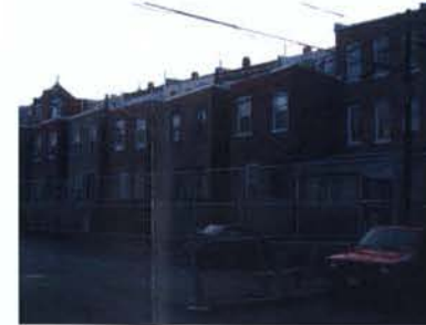
22nd Street Context - adjacent to site
