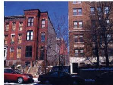
Existing Adjacent Buildings on F Street
