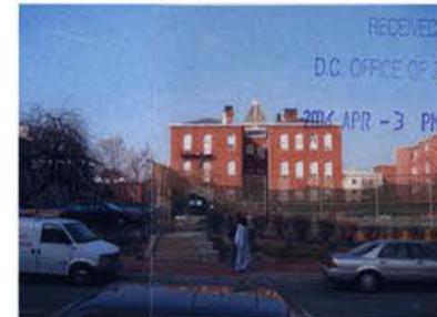
South facade from F Street
