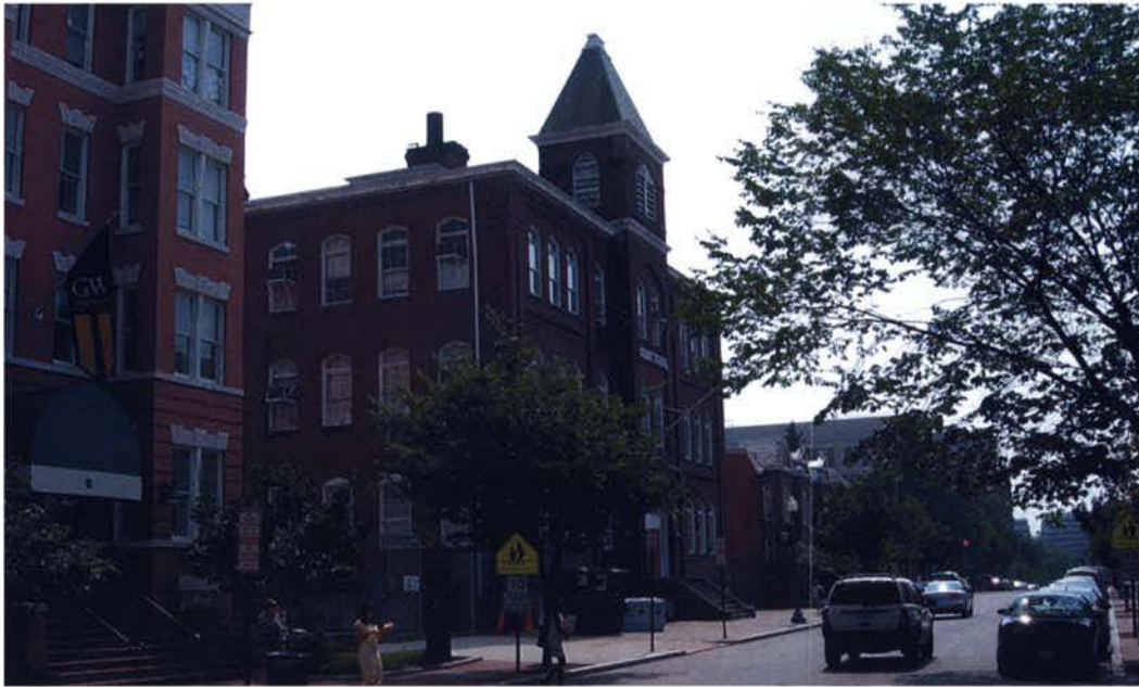
G Street and SWW from East
