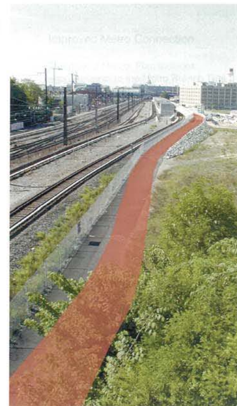
VIEW FROM NEW YORK AVENUE BRIDGE
