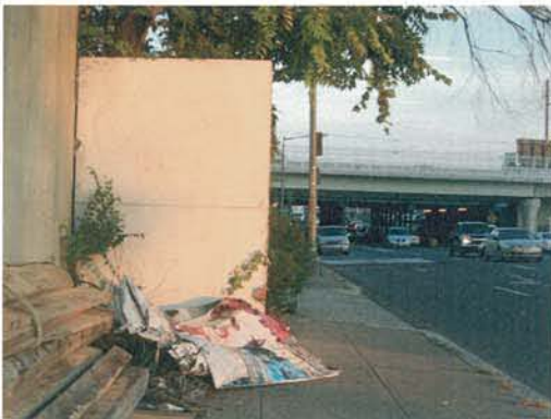
Existing Condition at Florida Avenue
