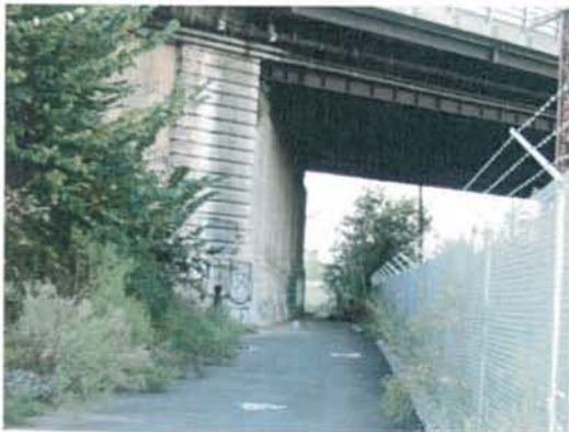
Existing Change of Grade at New York Avenue
