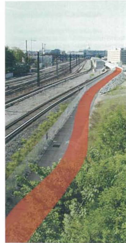
VIEW FROM NEW YORK AVE. BRIDGE
