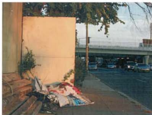
Existing Condition at Florida Avenue
