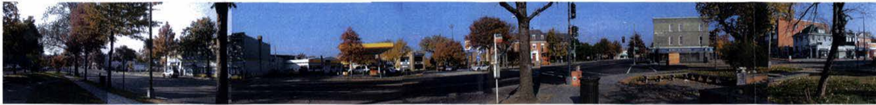
4 GEORGIA AVENUE ← SITE → GEORGIA AVENUE
