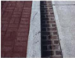
GRANITE CURB & BRICK GUTTER
