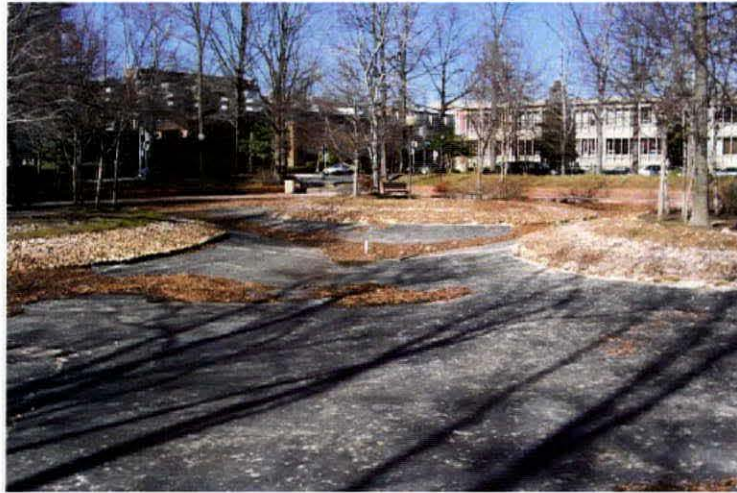
Figure 6 Pond basin - January 2006
