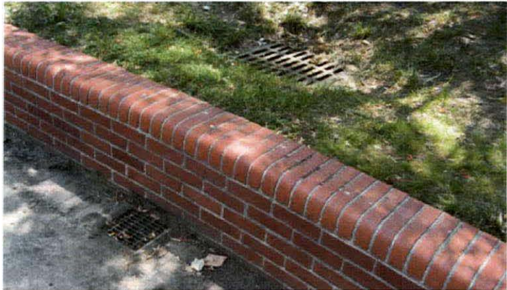
Figure 9 Area drain surrounded by dirt and debris
