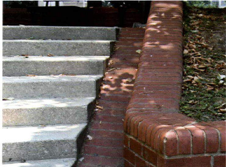
Figure 1 Brick runnel and concrete steps
