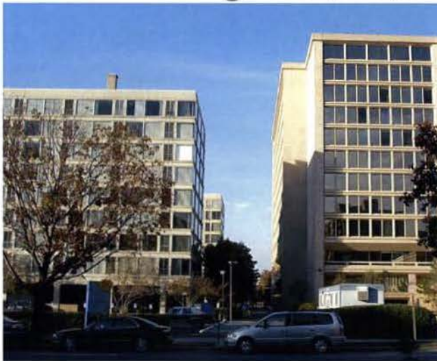
② View of Alley Looking North
