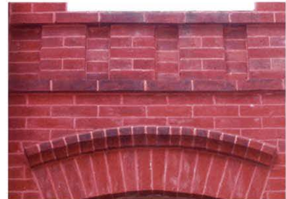
Recessed and projecting brick texture creating a play of light and shadow.
