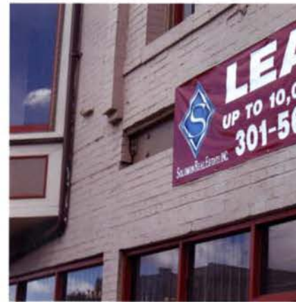
Painted metal channel with exposed fasteners
