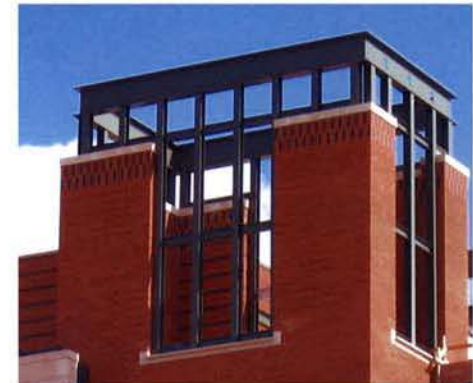
Dark painted metal frame with brick piers at Senate Square tower
