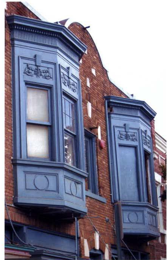
Metal panel and glass projected bays
