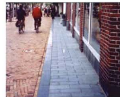
Bluestone border with brick paving
