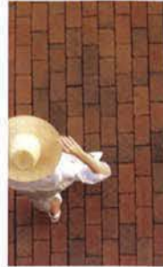
TYPICAL BRICK PAVEMENT
