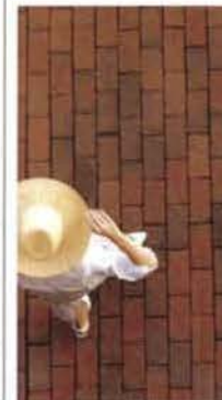
TYPICAL BRICK PAVEMENT
