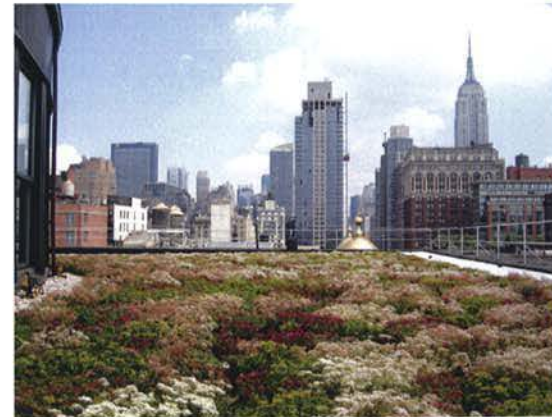
Cook+Fox Architects Office Green Roof New York, NY
