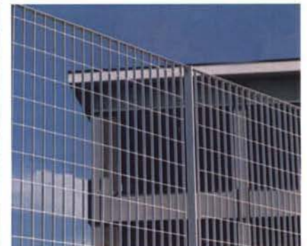
STEEL FENCE at EXISTING PARKING AREA
