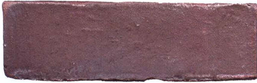
3RD ST FACADE BRICK
