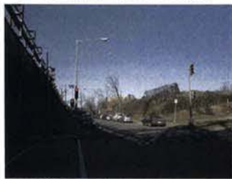
INTERSECTION OF 2ND STREET AND K STREET, N.E.
