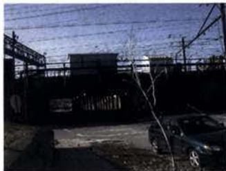
UNDERPASS AT 2ND STREET AND L STREET, N.E.
