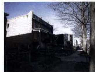
VIEW LOOKING NORTHEAST ALONG 3RD STREET, N.E.
