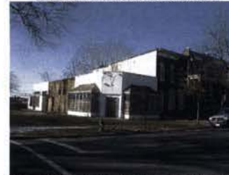
VIEW LOOKING NORTHWEST AT THE CORNER OF K & 3RD ST.
