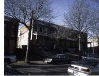
ABANDONED TOWNHOUSES TO BE DEMOLISHED
