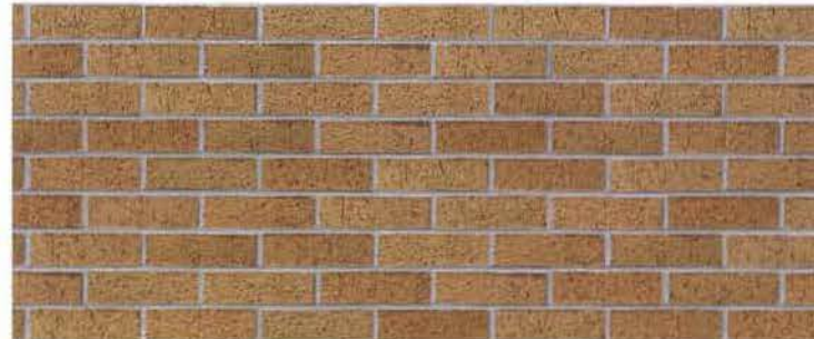
BRICK AT UPPER RESIDENTIAL UNITS
