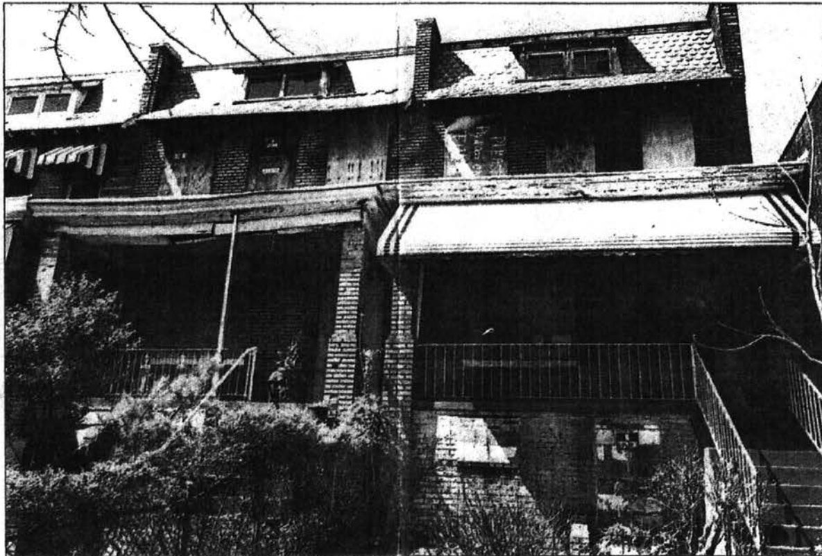
1020, 1022 and 1028 Third St. NE: Three abandoned properties in the Eckington neighborhood mar an otherwise tidy block. DCRA says 1020 and 1022 may not be attractive vacant properties but are secure, as required by city codes. Last October, DCRA referred 1028 to the Board of Condemnation for possible demolition.
