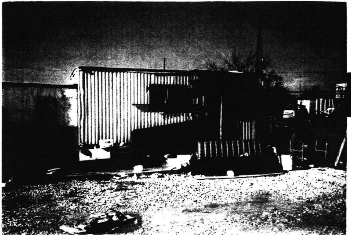
Front of Building Used As An Office / East Side
