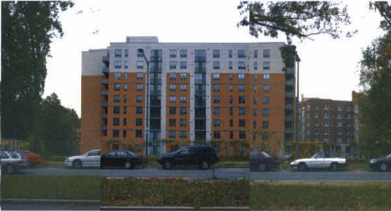
VIEW OF SITE WITH 3883 CONNECTICUT BEYOND.
