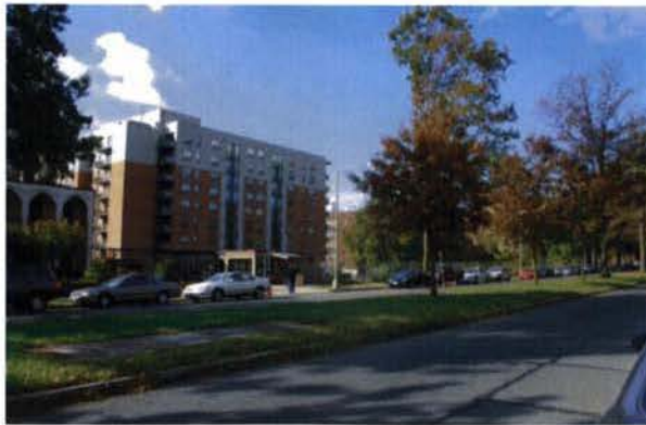
FROM TILDEN STREET LOOKING SOUTHWEST TOWARDS SITE
