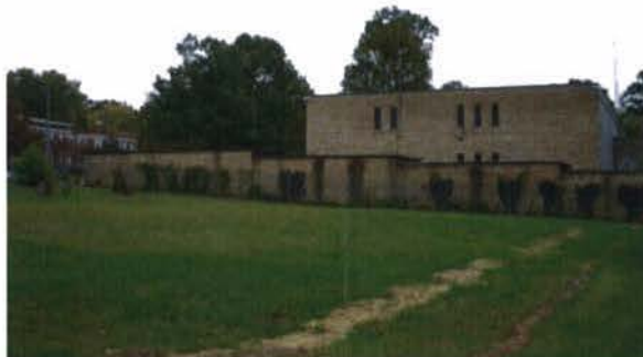
FROM SITE LOOKING EAST
