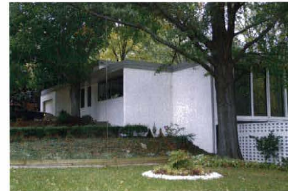
TILDEN STREET - SINGLE FAMILY HOUSE
