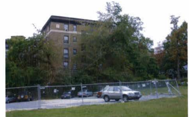
FROM SITE LOOKING WEST
