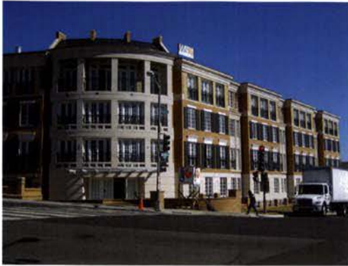
2501 WISCONSIN AVENUE NW
