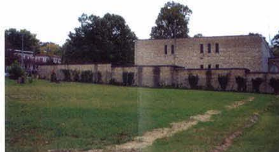
FROM SITE LOOKING EAST
