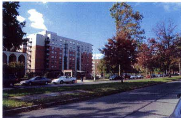
FROM TILDEN STREET LOOKING SOUTHWEST TOWARDS SITE
