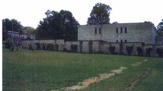
FROM SITE LOOKING EAST
