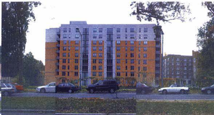
VIEW OF SITE WITH 3883 CONNECTICUT BEYOND.
