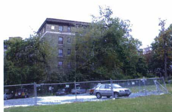
FROM SITE LOOKING WEST
