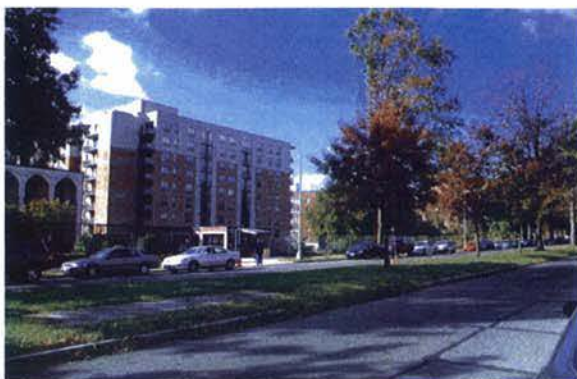
FROM TILDEN STREET LOOKING SOUTHWEST TOWARDS SITE
