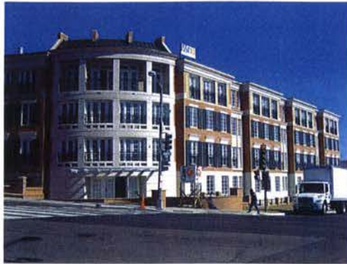
2501 WISCONSIN AVENUE NW
