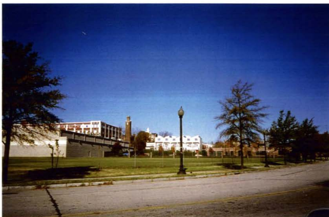
VIEW OF PROPERTY ALONG NORTHBOUND HARRY THOMAS WAY
