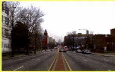
North Capitol Street, Before
