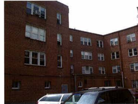
EXISTING EAST ELEVATION PHOTO
