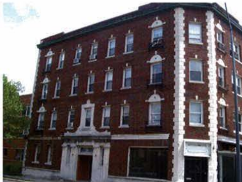
EXISTING NORTH ELEVATION PHOTO
