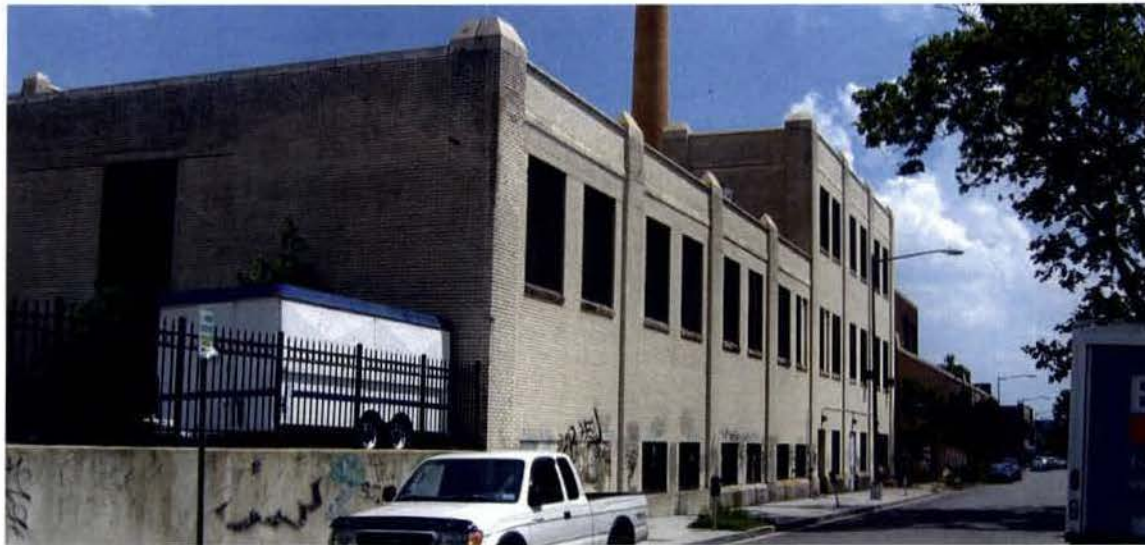
8th Street Facing Southeast
