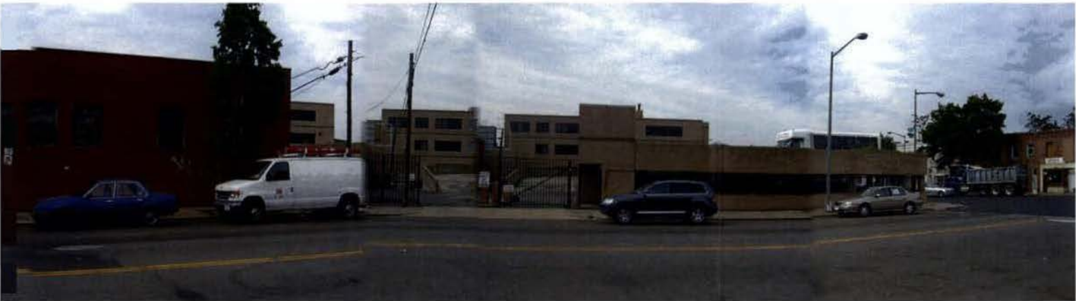
V Street Facing South
