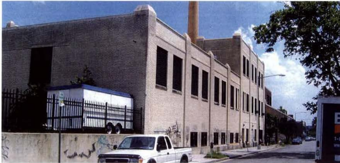
8th Street Facing Southeast
