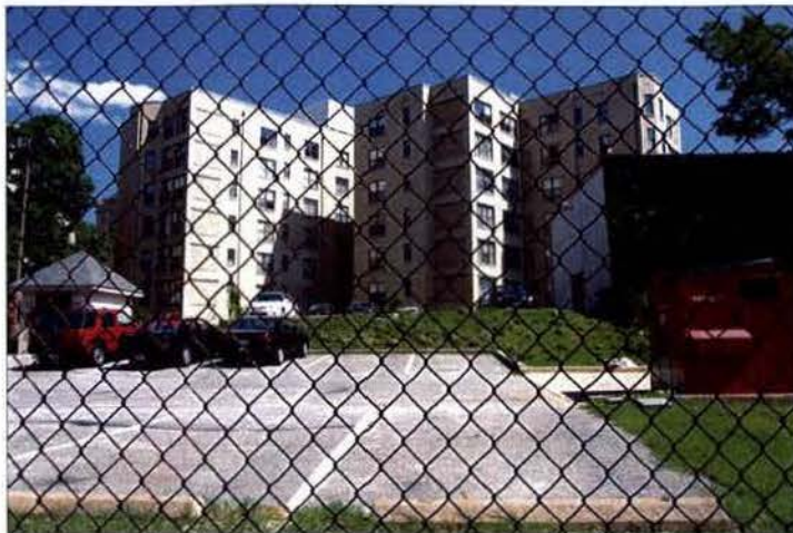
KALORAMA ROAD LOOKING SOUTH, ACROSS THE STREET FROM DORCHESTER HOUSE
