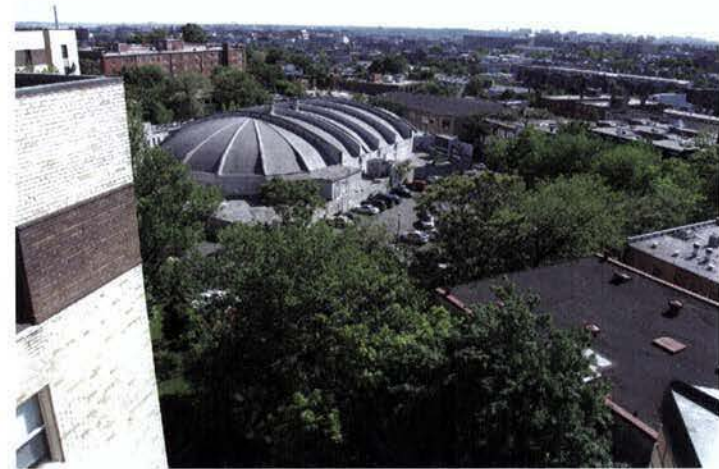
SITE FROM ROOF OF DORCHESTER HOUSE APARTMENTS (LOOKING SW)
