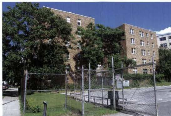
SOUTH SIDE OF KALORAMA ROAD (LOOKING EAST)
