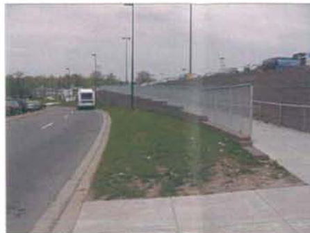
E EXISTING ADA RAMP PROVIDES OF PEDESTRIAN CONNECTION TO WEST SIDE OF ADJACENT "BIG BOX" SHOPPING CENTER.
