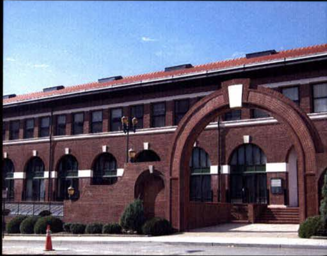
Railway Express Building: brick arches with limestone accents
