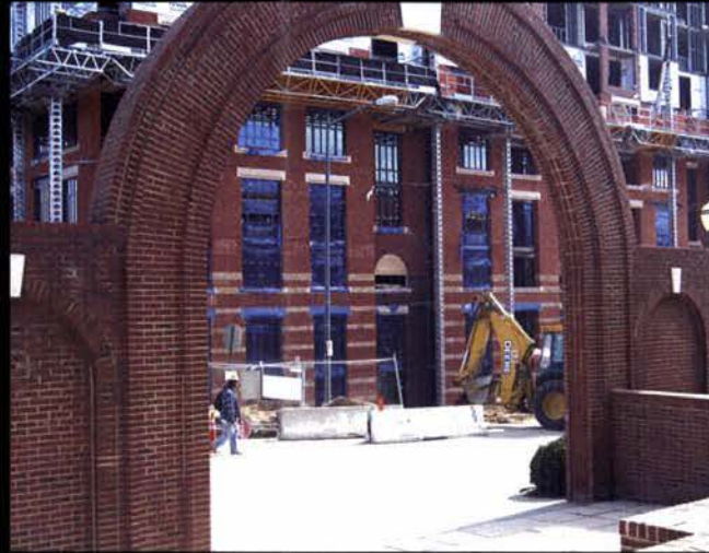
View from Railway Express Building across 2nd Street to project beyond; illustrates compatibility of refined brick palette and arched window design
