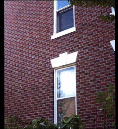
Neighboring townhouses: Flemish bond brick with dark accents
