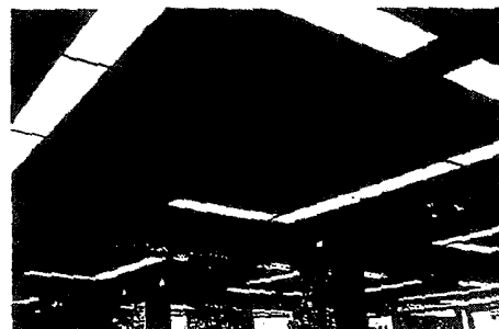
Cleveland Park Library Branch Inadequate Lighting
