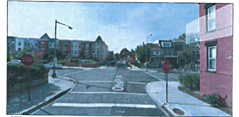
OTIS AT 11TH LOOKING WEST
